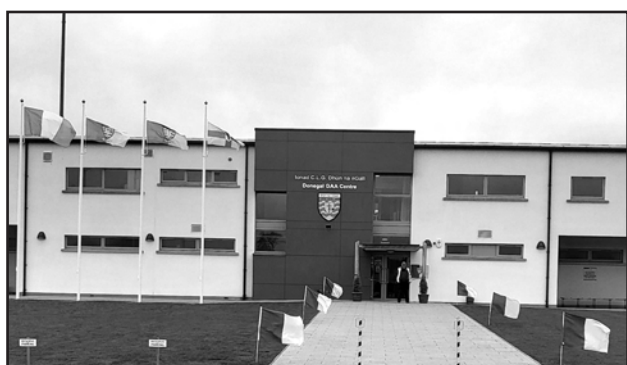
Opening of Donegal GAA Centre - Entrance
